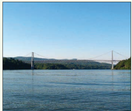
View of Bear Mountain Bridge (Town of Cortlandt)
