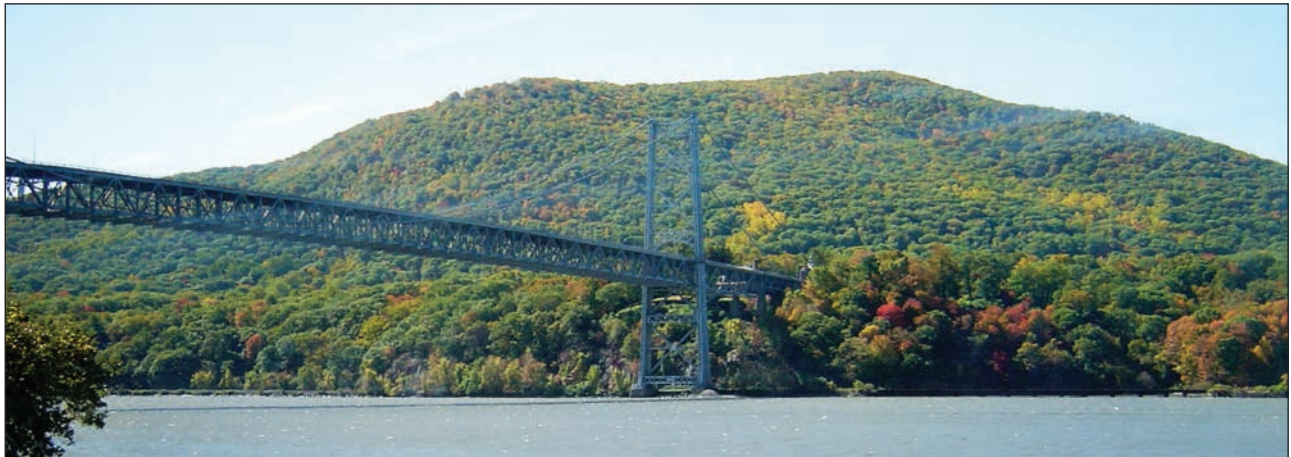
Bear Mountain Bridge (Town of Cortlandt)
