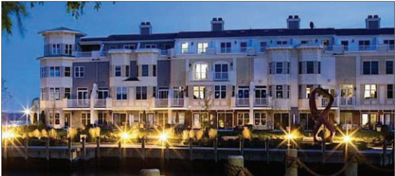
Example of Waterfront Residential Development (GDC, LLC.)
