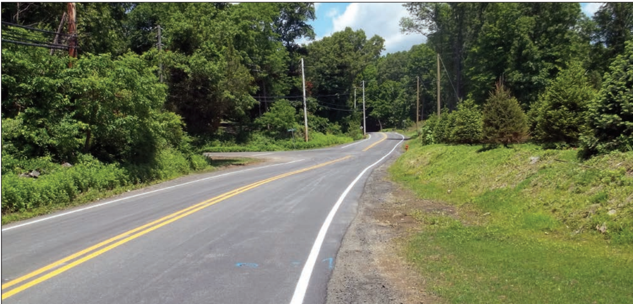
Furnace Dock Road (Town of Cortlandt)
